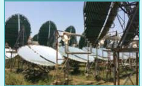
arranged where cooking is done with steam that is generated by solar collectors. Also students got deep knowledge of biogas plant. Air conditioner is also operated by steam that is generated by collectors.
